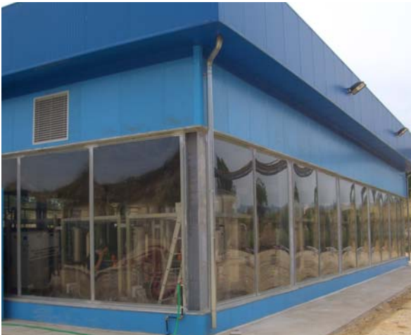
Location for leachate distillation
