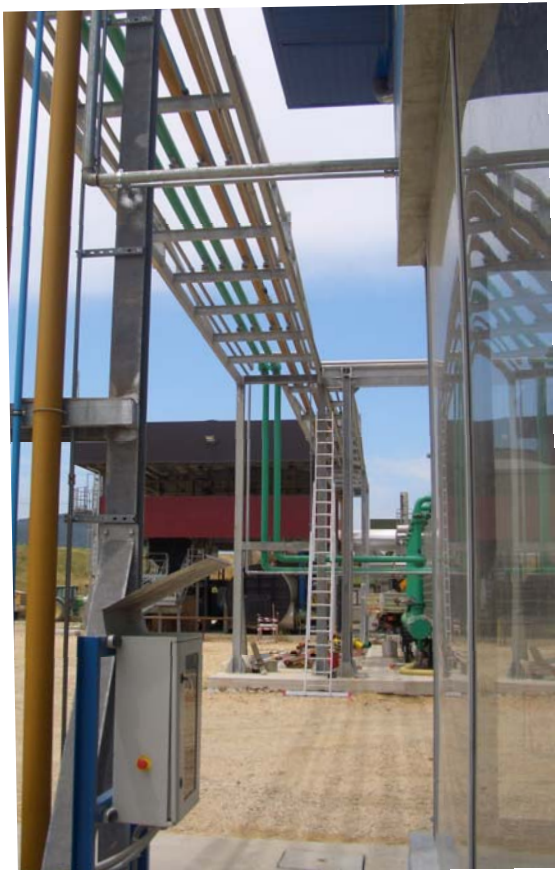
System of hot and cold water alimentation
